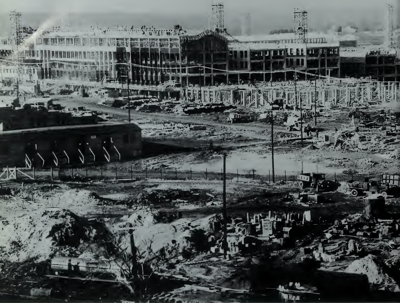
Section A progress, January 1942
